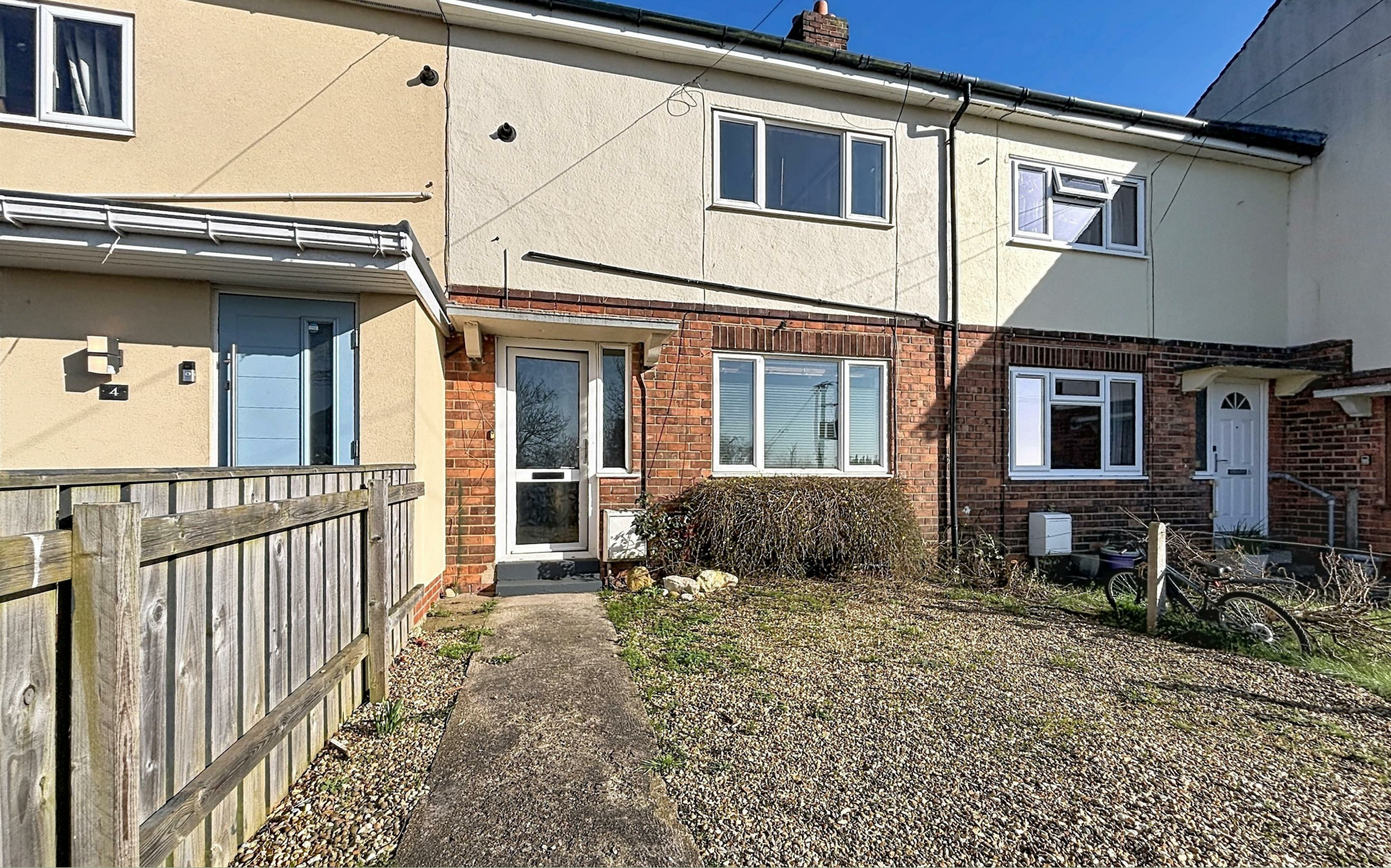
5 Holderness Cottages Arnold Lane West, Hull, HU11 5HS
